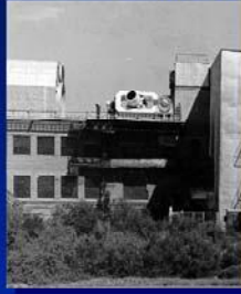
LE-1 laser radar building
