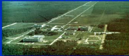
“Raduga” laser test range facility
