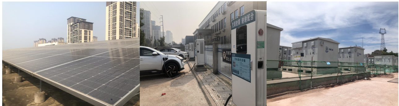
Figure 2. Integrated operation project of light storage and charging.
