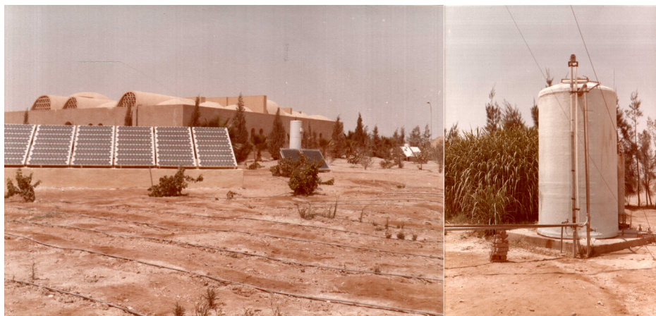
Fig. 5 The beginnings of solar pumping for agricultural irrigation in Egypt at Desert Development Center's research station in Sadat City in 1982. (a) Complete system and (b) tank with irrigation pump (source: CARES, formerly the Desert Development Center, The American University in Cairo).
